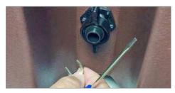
Locate the metal C-ring and with a small metal screwdriver, carefully slide it out of its groove on the spout end.
