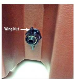
Turn the wing nut CLOCKWISE to loosen (reverse thread) until the faucet comes out.
