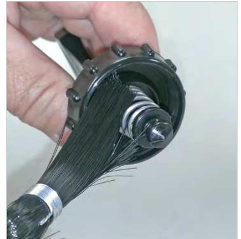
Clean the coil area on the faucet lever stem as well as around the inside area of the lever cap.
