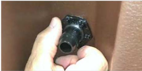
Using a **CLOCKWISE** or right-turn motion, screw back on the hex nut.
